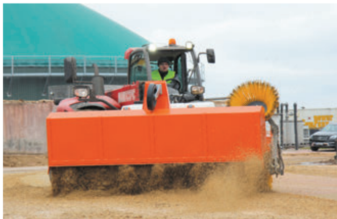
Free sweeping on a Biogas plant with the bema 75 Dual PowerMaster
