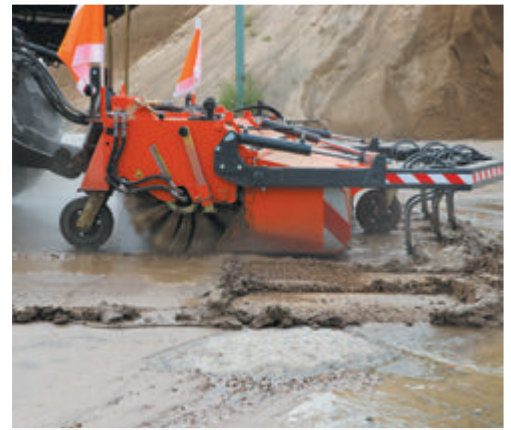
Scraping and rinsing with high-pressure
